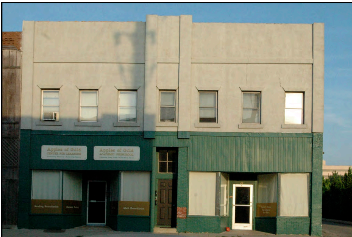
View of the resource, looking west across W. 2 nd St. N.
