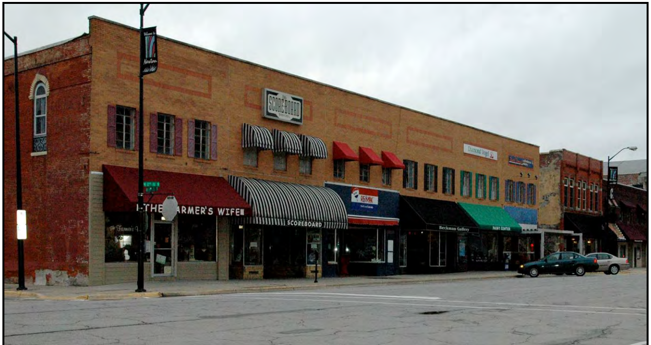
View of the building (first on left) looking northeast across N. 2nd Ave. W.
