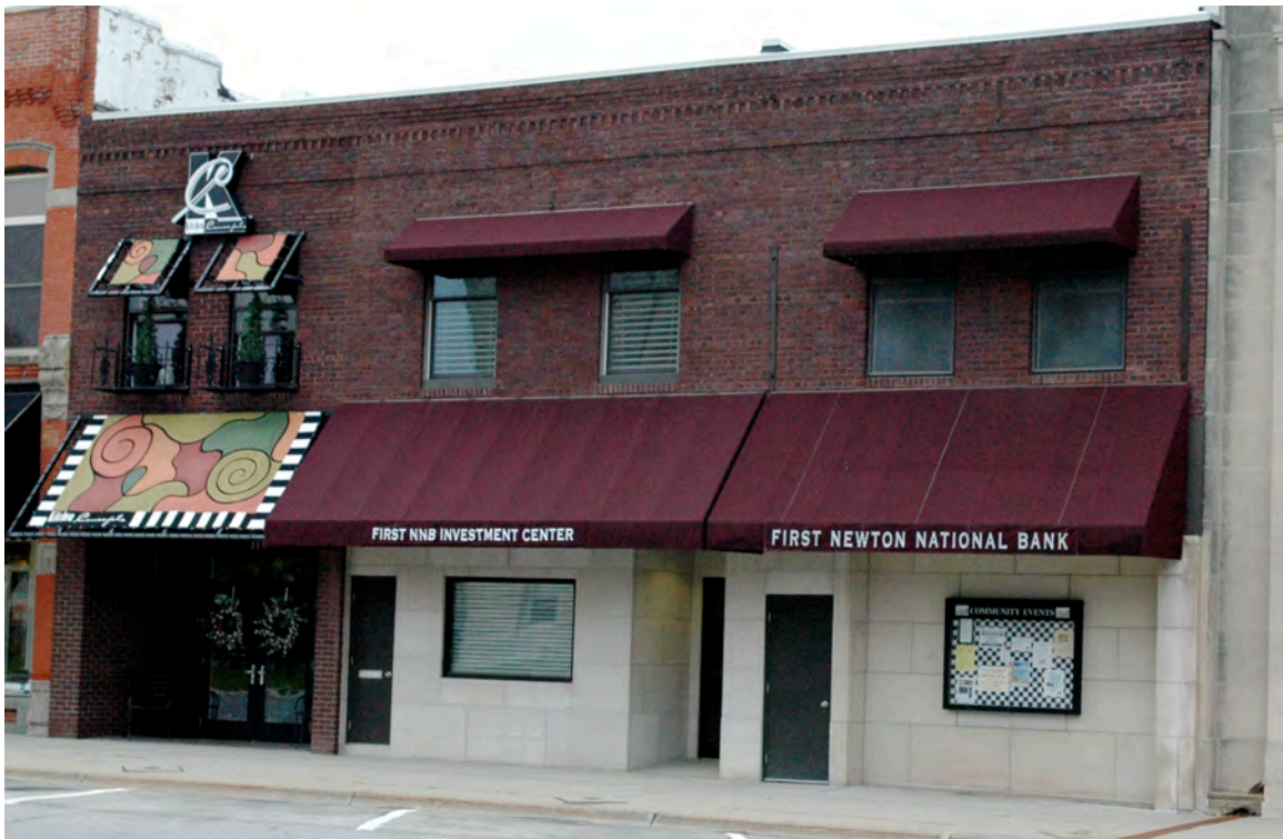
View of the resource, looking northwest across N. 2 nd Avenue W.
