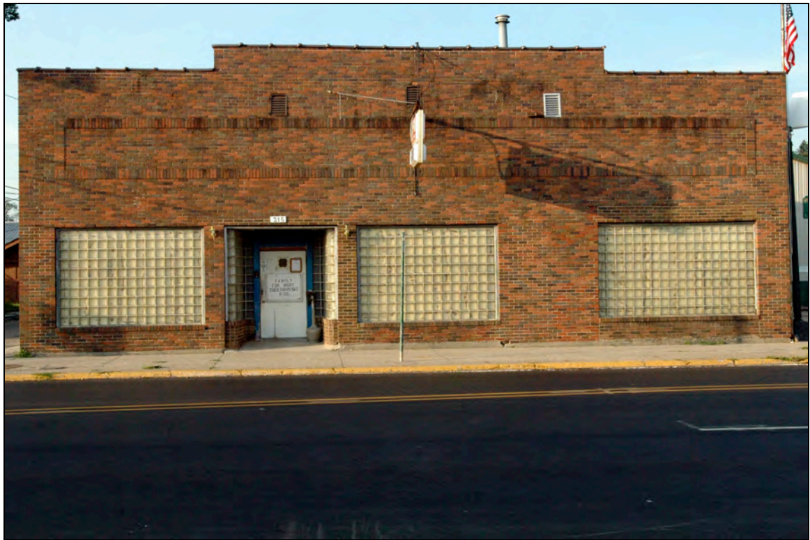
View of the building façade, looking south across 1 st Ave. W.
