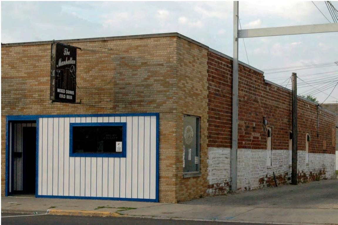
This photo of the structure's secondary façade shows the color of the original brick, as well as the replacement skin of lighter brick. In an effort to prevent vandalism during overnight hours, many owners of buildings with an alley frontage have painted the bottom portion of their building white.
